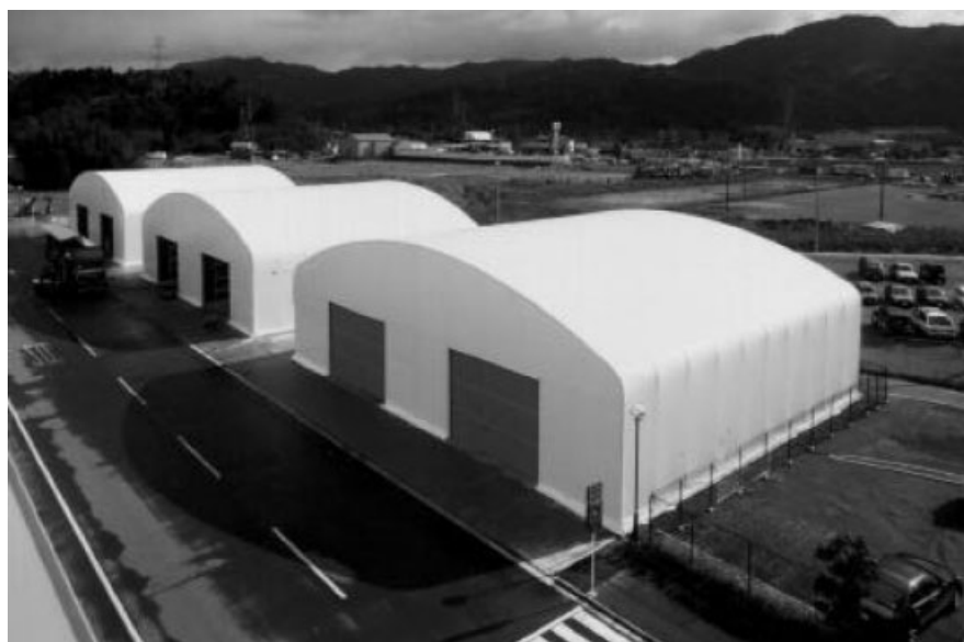
Fig. 19 Photograph of a temporary storage structure made from \text{TiO}_2 -treated tarpaulin (courtesy of Taiyo Kogyo Corp.).
